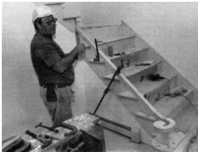
Figure 10. McLearn sets the rail assembly directly on the treads for marking the baluster holes in the underside of the rail. He uses a support block to align the volute directly above the newel hole in the starting step. He then transfers the baluster locations on the treads to the bottom of the rail with a combination square.
