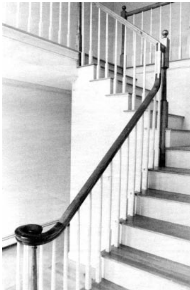
Figure 1. The handrail for this staircase starts with a spiral volute with an attached easement. The easement allows the volute to attach to the straight rail in an uninterrupted curve. At the top, another easement makes the transition into the gooseneck, which in turn butts into the landing newel.
