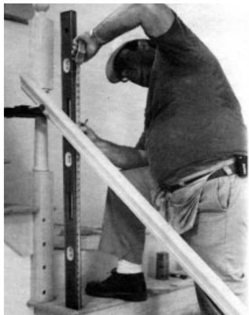
Figure 9. With the landing and starting newels in position, McLearn sets the straight rail in place, resting it on a clamp attached to the landing newel. He first sets the rail at the correct height, along a plumb line from the front edge of the top tread (left). Then holding the gooseneck in position so that its easement cut crosses the straight rail, he marks the cuts at the end of the straight section and at the top of the gooseneck (right).
