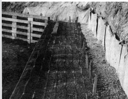
The Timberloc system relies on plastic "geogrid" to stabilize the slope. The first timber course (a) is stapled to a 4-foot-wide roll of geogrid material with pneumatically driven stainless-steel staples (b). Next, the geogrid is pretensioned with stakes (c) and is ready for a lift of backfill. The completed 6-foot wall (d) will have plantings in the open sections on the wall's face.
