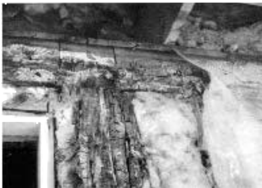
High moisture penetrated the exposed timbers on the interior (above, left) and condensed under the foam sheathing on the exterior. With the foam removed, decay in the sheathing and timbers became apparent (left). One corner post (above) had only 2½ inches of solid wood remaining.
