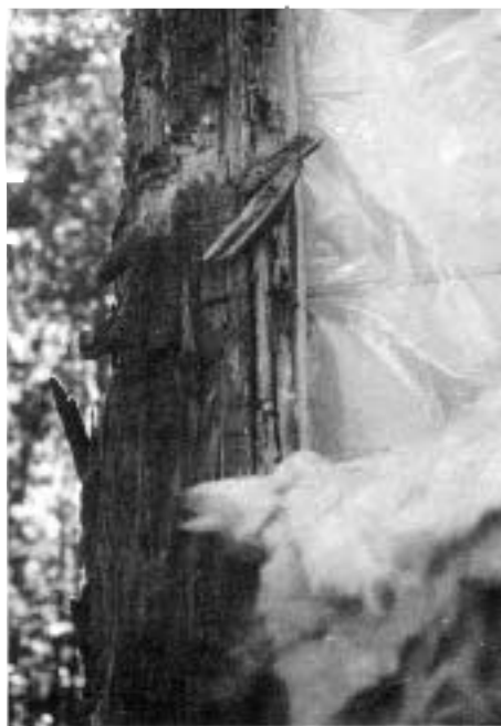
High moisture penetrated the exposed timbers on the interior (above, left) and condensed under the foam sheathing on the exterior. With the foam removed, decay in the sheathing and timbers became apparent (left). One corner post (above) had only 2½ inches of solid wood remaining.
