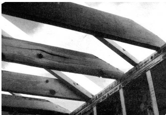
Figure 7. Overtapering joists to fit beneath roofs creates inadequate joist depth at the plate. A proper cut (right) leaves at least half the depth of the joist.
