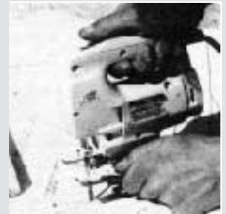
In place of a pattern marker, the author uses a jigsaw at slow speed to transfer a sink pattern to a countertop.
