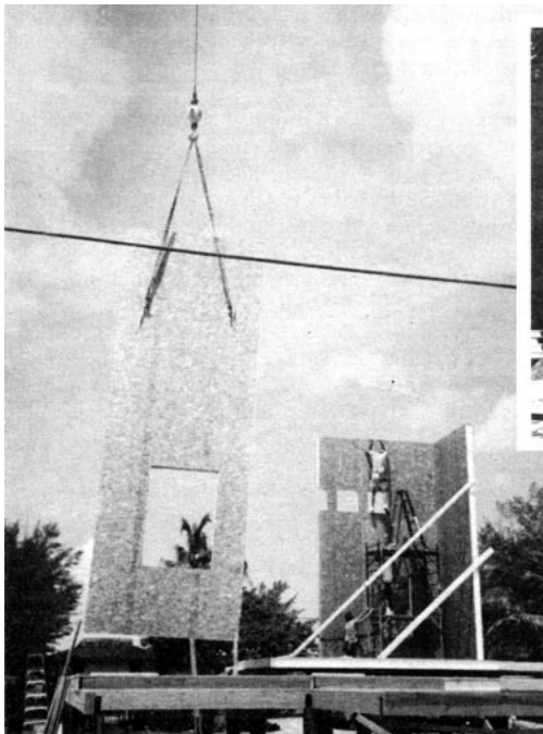
Heave ho! Placing large roof panels or two-story verticals usually requires a crane (left). But a strong crew can handle some large panels, like this gable end, above, without a crane.
