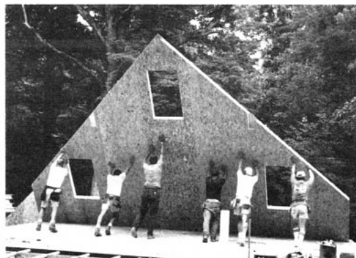
Heave ho! Placing large roof panels or two-story verticals usually requires a crane (left). But a strong crew can handle some large panels, like this gable end, above, without a crane.
