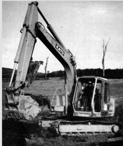
The excavator is the best all-round machine for residential site work.
