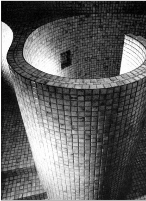
Figure 2. Util-i-Crete — a 1/4-inch-thick backerboard — can be bent around a 24-inch radius to form a curved tile wall, like this shower stall.
