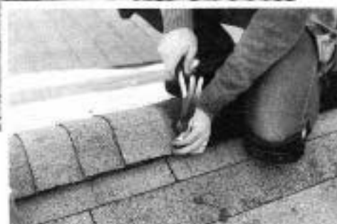
Low-profile ridge vents are capped with shingles to visually blend the vent with the rest of the roof.
