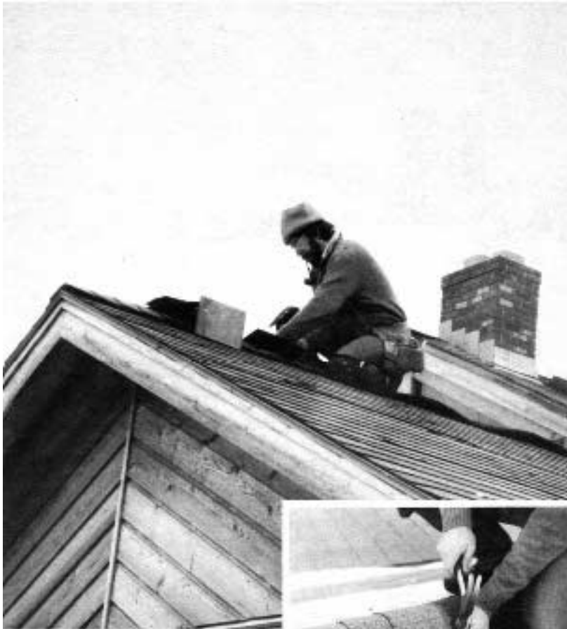
Low-profile ridge vents are capped with shingles to visually blend the vent with the rest of the roof.
