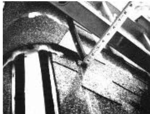
Figure 1. The extra layer of asphalt on architectural-type shingles can hold the edge of the vent off the roof, allowing rain and snow to blow in below the baffles. To remedy this problem, strip off the extra layer from the shingle and caulk along the bottom edge of the vent.
