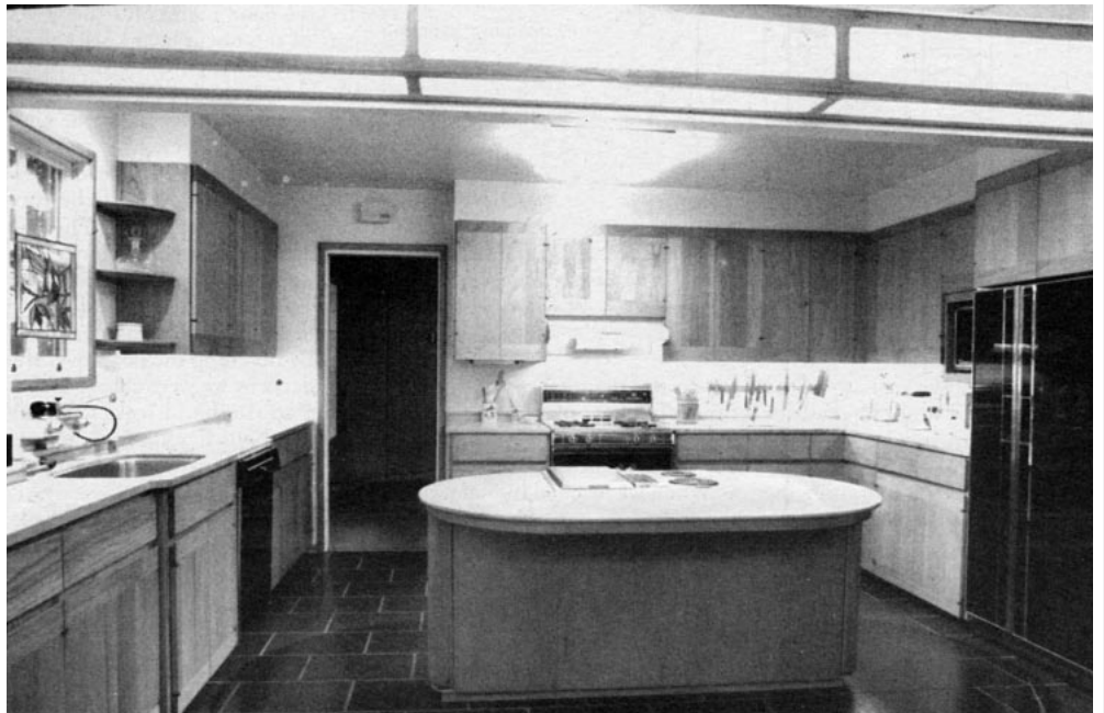
Incandescent ceiling lights and undercabinet fluorescents make the work areas in this kitchen bright and functional. A ceiling fluorescent fixture and valance lights (foreground) provide even, general lighting.
