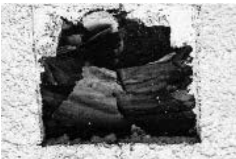
Figure 5. Moderate wetting will cause the facing of gypsum sheathing to delaminate. With increased wetting, the core will deteriorate, as seen in this cut-away section.
