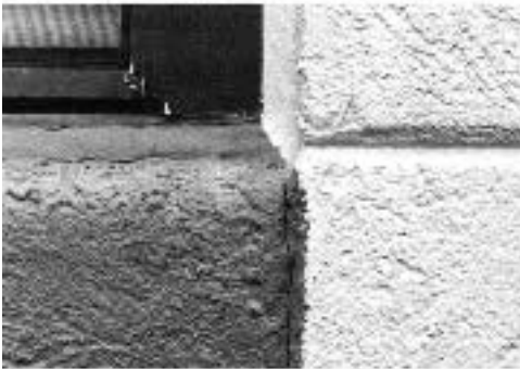
Figure 3. V-grooves, added for decorative effect, should never line up with window or door openings. This one cracked, was recoated with the manufacturer's elastomeric coating, and cracked again within a year.
