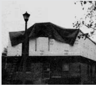
A house under wraps.
