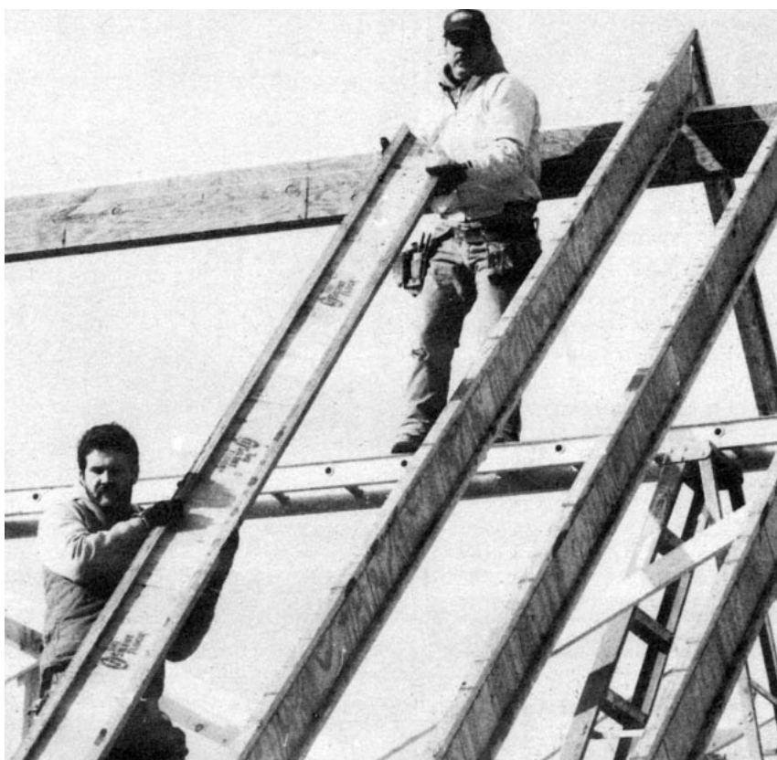
Two men can easily position a 24-foot I-beam rafter. The wood I-beams are lightweight and straight enough that they don't need crowning.
