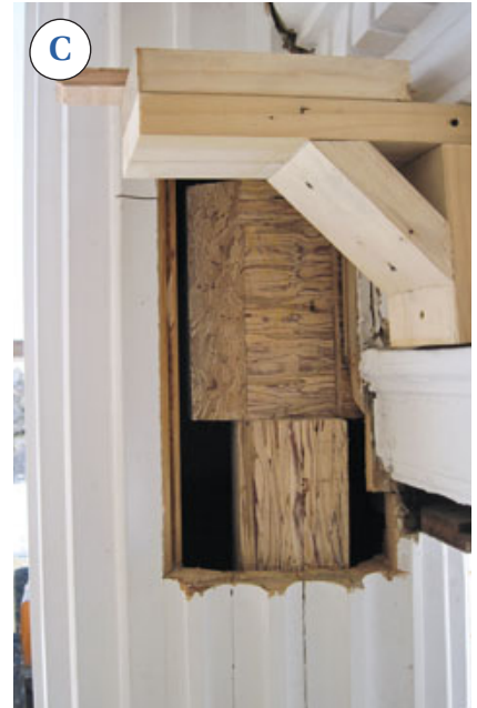
Figure 7. At the end of the colonnade, the carpenters used one of the old columns to practice scribing to the adjoining porch roofline (A). A plywood template helped in orienting the flutes to the existing trim (B). Where the support beam of the adjacent deck dies into the column, a recip saw (C) was used to create the beam pocket (D).
