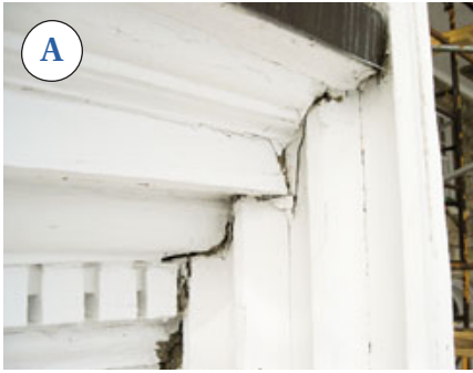
Figure 6. Replacing the columns at each end of the porch was complicated by scribed trim (A) and abutting rooflines (B). One of these columns also concealed a Parallam post that supported the end of a load-bearing beam (C, D).
