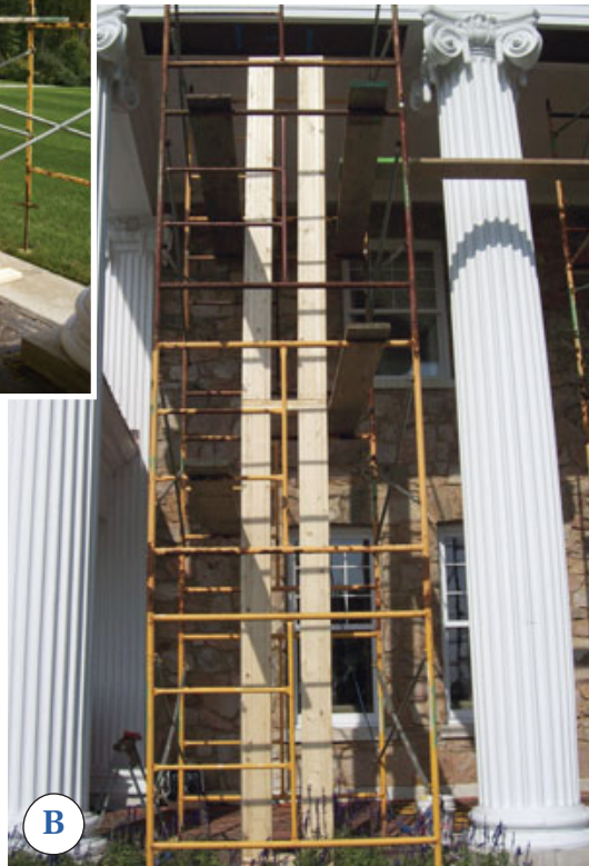
Figure 1. To temporarily support the porch roof while the columns were replaced, the carpenters built posts from 10-foot-long 2x4s and 2x6s (A). The double-post assemblies were joined by top and bottom plates stacked two high (B), then sheathed with 1/2-inch plywood (C). Full-length 2x4 strongbacks were added to the outside for rigidity.
