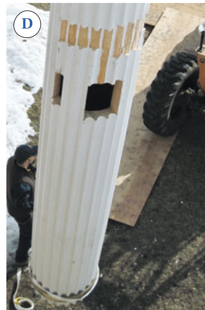
Figure 7. At the end of the colonnade, the carpenters used one of the old columns to practice scribing to the adjoining porch roofline (A). A plywood template helped in orienting the flutes to the existing trim (B). Where the support beam of the adjacent deck dies into the column, a recip saw (C) was used to create the beam pocket (D).
