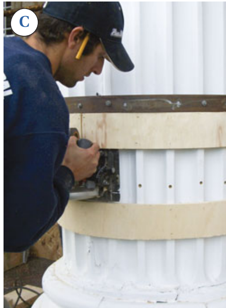
Figure 2. The original plan was to replace only the column bases. Accordingly, the crew installed structural steel clamp rings around the shafts (A) and shifted the weight from the pedestals to the concrete porch using 20-ton hydraulic jacks. Rings of bending plywood served to guide the cutting of the wood columns, which was done with reciprocating saws (B) and circular saws (C). Removing the bases (D) confirmed that the interiors were delaminating and that the columns would have to be replaced.
