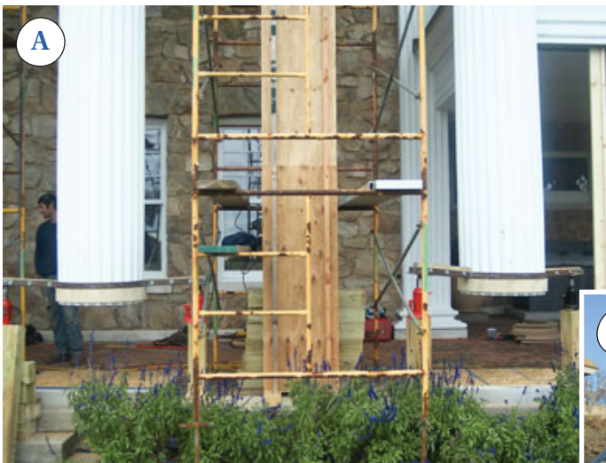
Figure 3. After cutting away the bases (A), the crew placed cribbing under the shafts (B) while awaiting the delivery of new columns (C).
