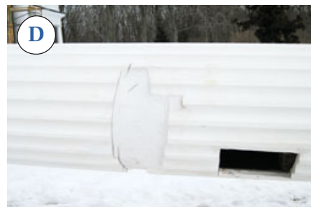
Figure 9. A round support pedestal (A) was built to replace the Parallam post in the old corner column. After carefully checking its final position on the porch (B), the carpenters slid the pedestal — dubbed “the plug” — into the column (C), where it was secured with lag screws driven from the outside. The raw wood of the scribed column was primed (D) before final installation.
