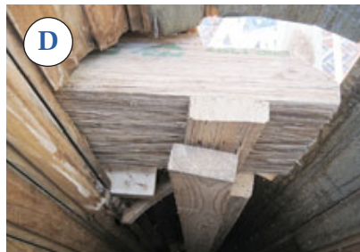
Figure 6. Replacing the columns at each end of the porch was complicated by scribed trim (A) and abutting rooflines (B). One of these columns also concealed a Parallam post that supported the end of a load-bearing beam (C, D).
