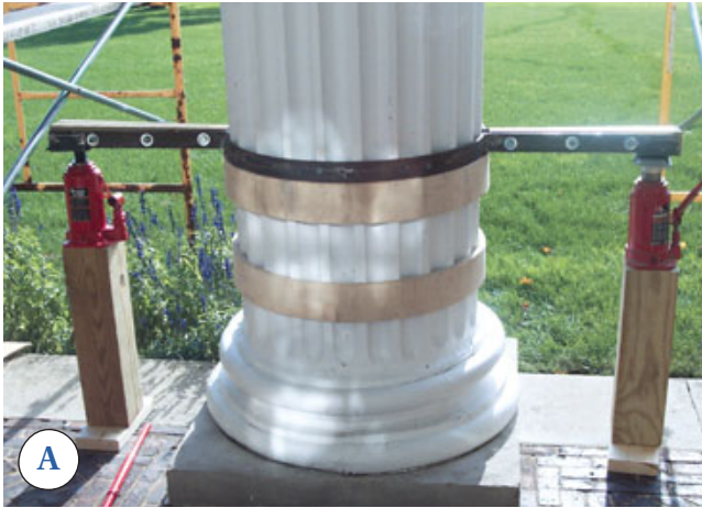
Figure 2. The original plan was to replace only the column bases. Accordingly, the crew installed structural steel clamp rings around the shafts (A) and shifted the weight from the pedestals to the concrete porch using 20-ton hydraulic jacks. Rings of bending plywood served to guide the cutting of the wood columns, which was done with reciprocating saws (B) and circular saws (C). Removing the bases (D) confirmed that the interiors were delaminating and that the columns would have to be replaced.
