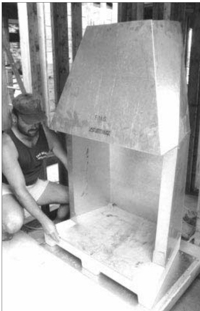
A worker installs the metal shroud of a Firecast masonry fireplace.
