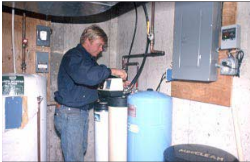
A subcontractor installs a water-softening system to treat all incoming water.
