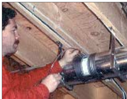
Figure 3. A flow station (left) and magnehelic gauge (center) are used to measure air flow and static pressure in the duct system. To balance the intake and exhaust sides, the installer adjusts in-line dampers (right).
