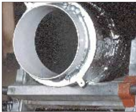
Figure 2. The author uses double-ducted collars (left) to seal the outside vapor barrier of insulated flex duct to the exterior intake and exhaust hoods. He applies a bead of sealant around the collar before attaching it to the band joist (right).
