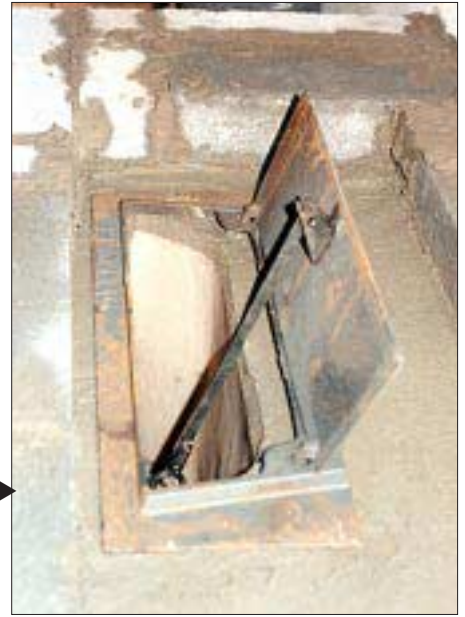
▶ Figure 4. The cast-iron damper mounts directly on top of the curved throat component.
