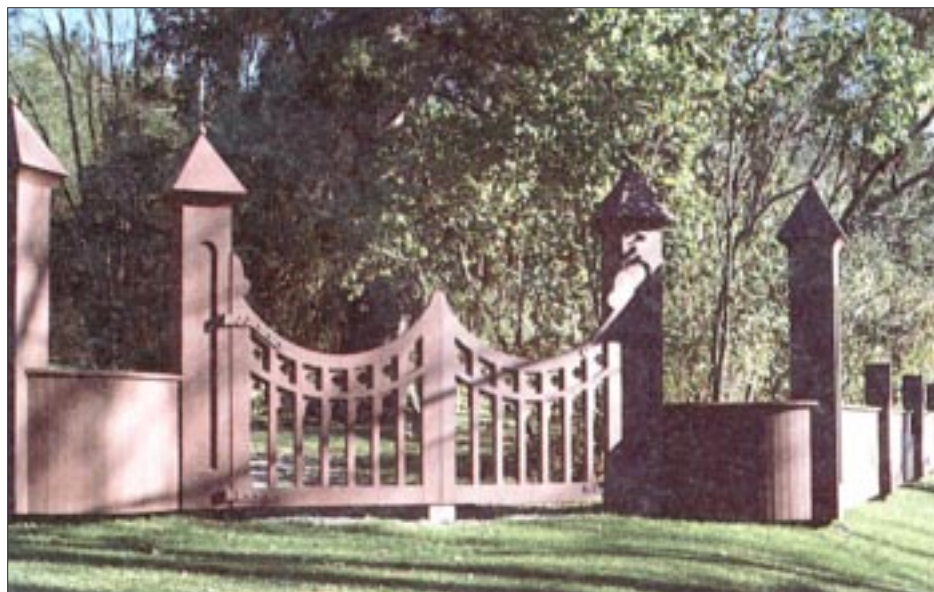
Builder Blake Spencer used historical photos to work out the details of the historic fence restoration at the Morrill Homestead in Strafford, Vt. The main gate is the kind you would imagine passing through on the way to meet St. Peter. Or Walt Disney.
