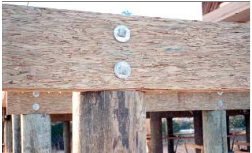
Figure 2. The gas-powered chain saw is the weapon of choice for notching pilings (above). Girders are tacked in place for drilling the bolt holes (above right). The author likes treated Parallam girders (right) because they come in long lengths, making them quicker to install than built-up girders.
