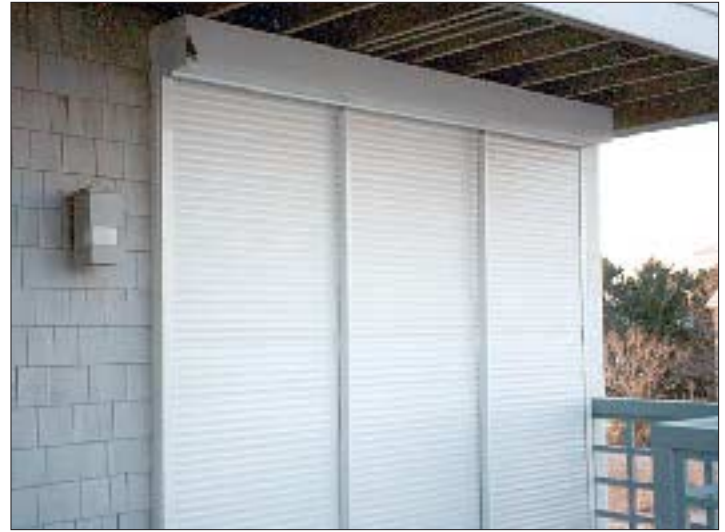
Figure 6. Coastal builders must take special care to seal openings against wind-driven rain. To install a window (left), the housewrapped opening is first covered with tar paper. The window is then installed in a bed of caulk. The author uses only clad windows rated for coastal conditions. The author recommends storm shutters (right) for all coastal homes to prevent hurricane winds and flying debris from bursting the glass in windows and doors.
