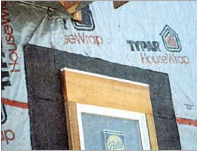
Figure 6. Coastal builders must take special care to seal openings against wind-driven rain. To install a window (left), the housewrapped opening is first covered with tar paper. The window is then installed in a bed of caulk. The author uses only clad windows rated for coastal conditions. The author recommends storm shutters (right) for all coastal homes to prevent hurricane winds and flying debris from bursting the glass in windows and doors.
