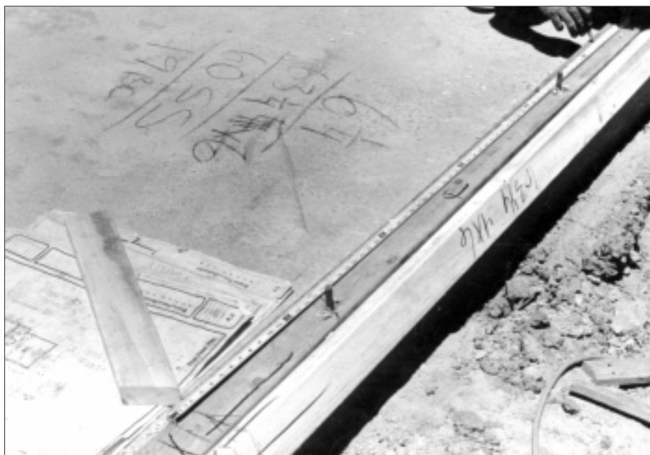
Figure 4. The author details king studs with an X. The line coming off the X indicates the direction of the header. Note the details written in large numbers on the slab, which give the cutting list for that window package.
