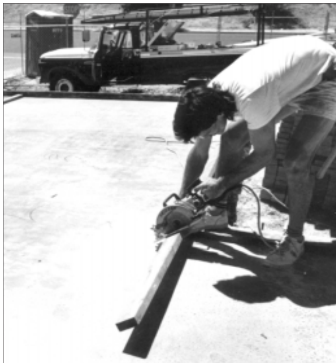
Figure 3. Plating goes quickly because the author leaves his tape measure in his belt and makes end cuts by eye from the chalk lines.
