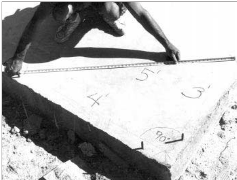
Figure 1. The author begins layout at the two longest exterior walls that form an outside corner. He measures in a stud width from the edge of the slab and snaps a line along the longer wall. Then, using the 3-4-5 triangle method, he lays out the adjoining wall at exactly 90 degrees. He measures the other walls from these two, to create a perfectly square layout.
