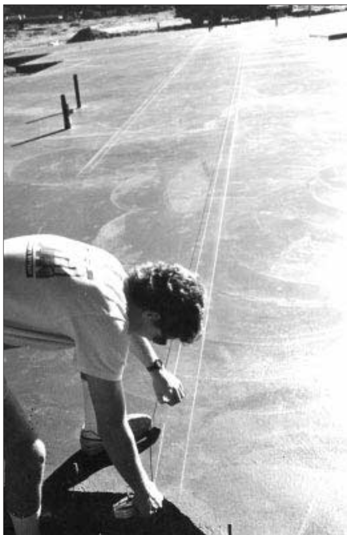
Figure 1. The author begins layout at the two longest exterior walls that form an outside corner. He measures in a stud width from the edge of the slab and snaps a line along the longer wall. Then, using the 3-4-5 triangle method, he lays out the adjoining wall at exactly 90 degrees. He measures the other walls from these two, to create a perfectly square layout.
