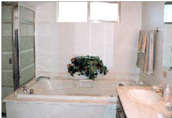
Cultured marble products are now widely available in a variety of colors and styles. In this bathroom, the shower walls, whirlpool surround, and vanity top are all cultured marble.
