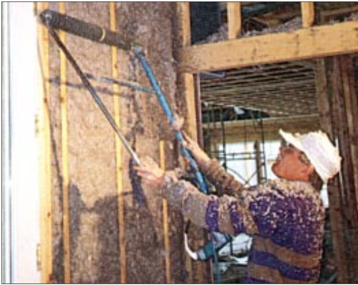
Figure 2. Excess cellulose or “overspray” is removed with a scrubber (left). Powered by an electric drill, the scrubber’s spiral groove brush creates a smooth face even with the plane of the wall studs. The excess material is swept up (right) and sent back through the hopper to be blown onto the next wall.
