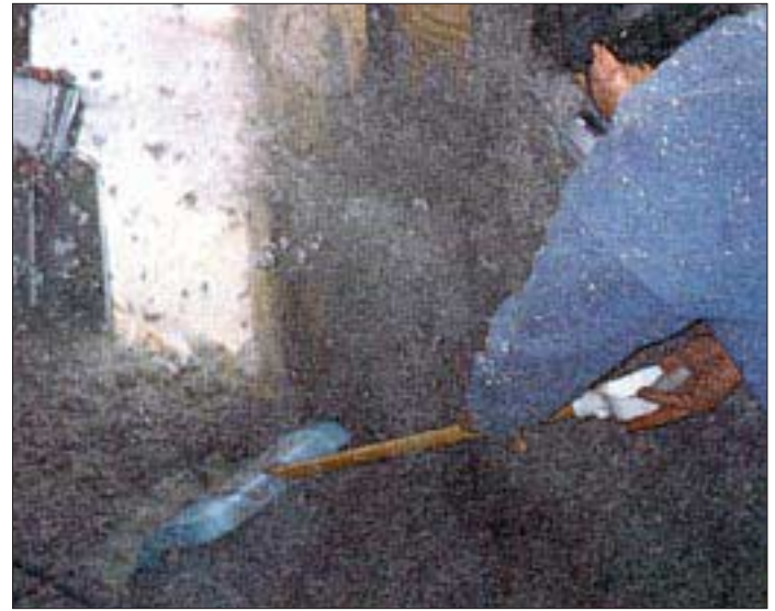
Figure 2. Excess cellulose or “overspray” is removed with a scrubber (left). Powered by an electric drill, the scrubber’s spiral groove brush creates a smooth face even with the plane of the wall studs. The excess material is swept up (right) and sent back through the hopper to be blown onto the next wall.
