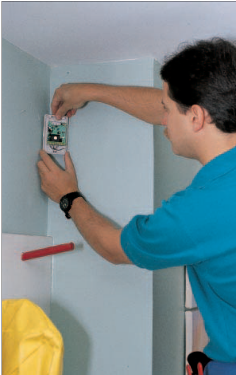
A home-security contractor installs an AT&T wireless infrared detector.
