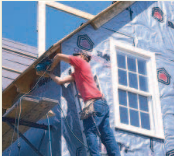
Proper staging and good planning are keys to reducing fall risks.
