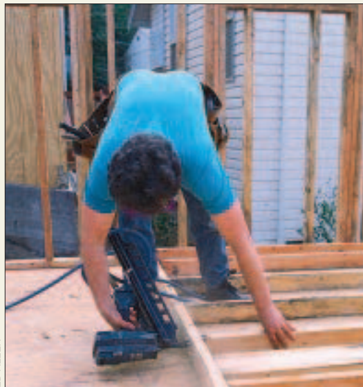
To reduce nail-gun injuries, wear eye protection and have stable footing.
