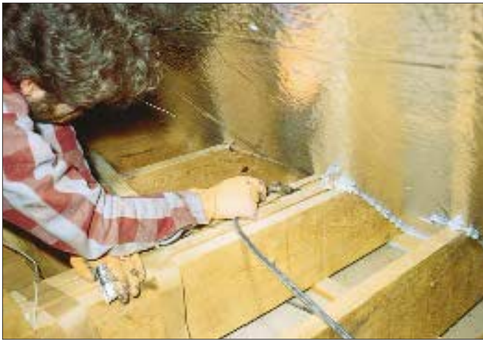
Figure 2. In existing structures, foil-faced foam provides an effective air barrier behind knee walls. Here, spray foam seals the gaps left where the foam board has been installed over unfaced batts between the rafters.
