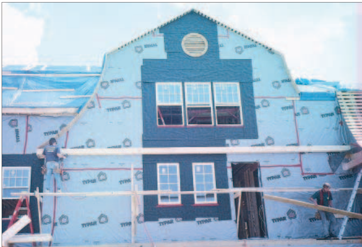
To protect this oceanfront home from wind-driven rain and surf spray, the builder has covered the housewrap around doors and windows with a self-adhering bituminous membrane.
