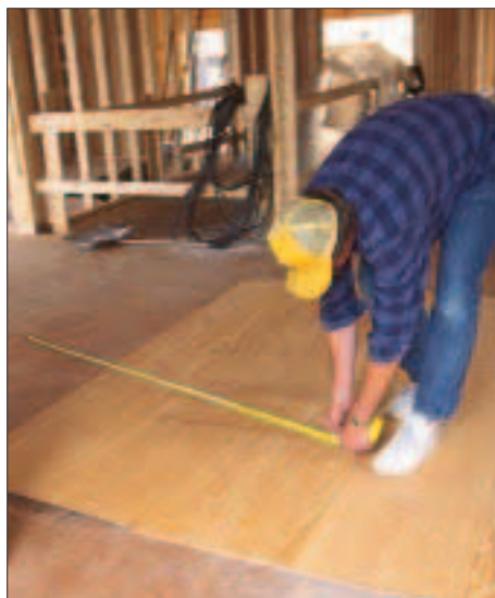
Figure 5. Roof sheathing layout. The author laid out and cut roof sheathing three pieces at a time by swinging radiuses from a pivot point that represented the top of the rafter (left and center). The plywood was nailed off, then cut square to the rafters in place (right).
