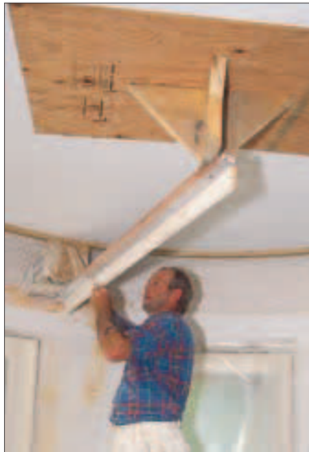
Figure 7. Interior trim. By swinging a sheet-metal screed from a pivot jig attached to the center point of the ceiling, the plasterer created a perfectly round crown molding (left). Wood baseboards and window casings (right) had to be steamed and clamped into place to make the bend.
