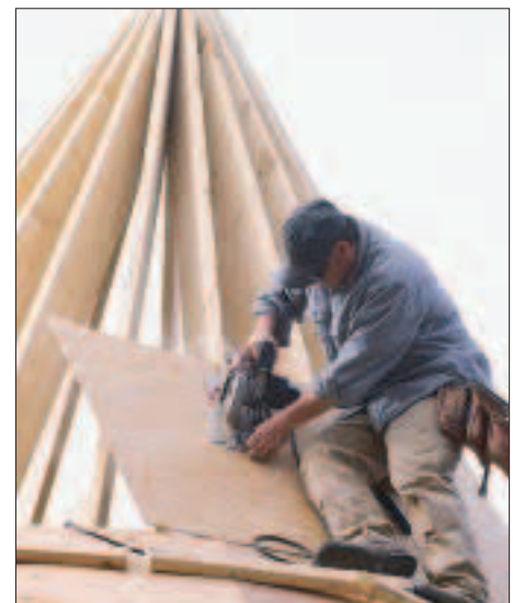
Figure 5. Roof sheathing layout. The author laid out and cut roof sheathing three pieces at a time by swinging radiuses from a pivot point that represented the top of the rafter (left and center). The plywood was nailed off, then cut square to the rafters in place (right).
