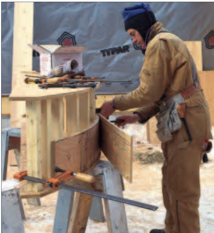
Figure 3. Curved headers. Carpenters made laminated window headers by bending three layers of \frac{1}{2} -inch plywood around a form, and gluing it and screwing it together (left). Each header has two triple-laminated pieces, joined at top and bottom by \frac{3}{4} -inch-plywood plate material (right).
