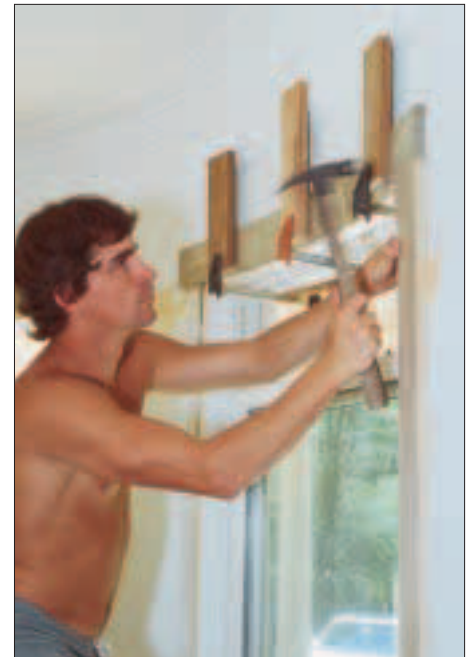
Figure 7. Interior trim. By swinging a sheet-metal screed from a pivot jig attached to the center point of the ceiling, the plasterer created a perfectly round crown molding (left). Wood baseboards and window casings (right) had to be steamed and clamped into place to make the bend.
