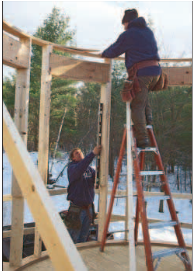
Figure 2. Plywood plates. A double layer of \frac{3}{4} -inch plywood formed the bottom plates of the round walls; the top plates took four layers.
