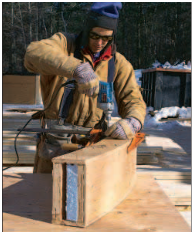
Figure 3. Curved headers. Carpenters made laminated window headers by bending three layers of \frac{1}{2} -inch plywood around a form, and gluing it and screwing it together (left). Each header has two triple-laminated pieces, joined at top and bottom by \frac{3}{4} -inch-plywood plate material (right).
