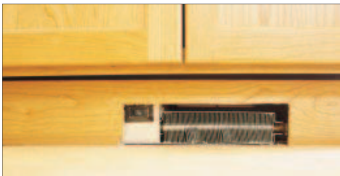
Figure 1. Hydronic kickspace heaters (above) require careful layout and plumbing to fit precisely in a base cabinet bottom (left).
