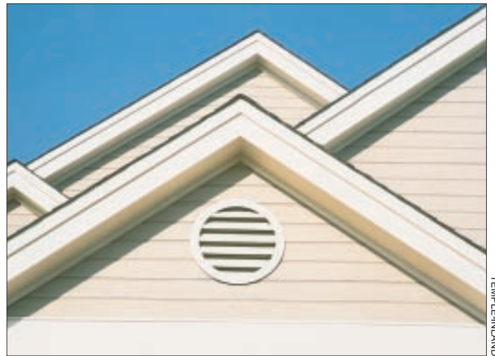
Figure 5. Hardboard trim, such as TrimCraft (left) and PrimeTrim (right), can be used for fascia, rake, and corner boards in combination with a variety of wood sidings.
