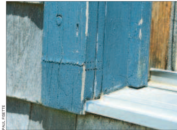
Figure 4. Differing grain orientation in the glued-up pieces can cause telegraphing at finger joints in brick molding (left) and at edge-glued joints in wide finger-jointed trim (right). To reduce problems, specify vertical-grain material and exterior glue, and keep the trim well painted.
