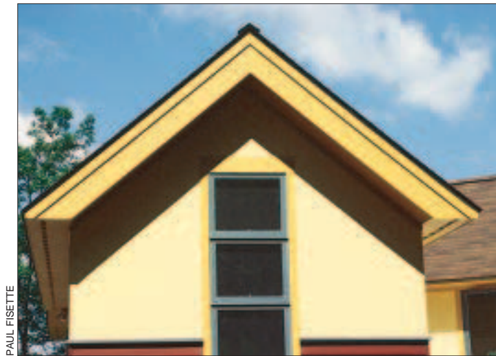
Figure 5. Hardboard trim, such as TrimCraft (left) and PrimeTrim (right), can be used for fascia, rake, and corner boards in combination with a variety of wood sidings.
