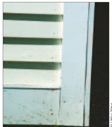
Figure 6. The most common problem with hardboard is swelling around nail heads and at the ends of boards. To reduce problems, paint all cut edges, caulk breaks in the surface at nail heads, and leave room at butt joints for expansion.
