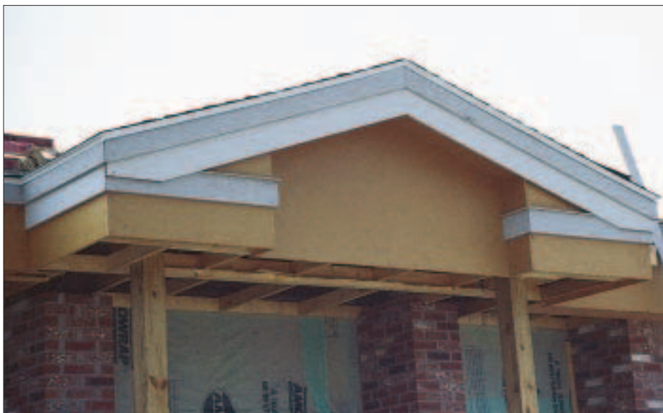
Figure 2. Combined with MDO plywood at wide soffits and deep rakes, LVL trim makes for a durable, seamless look.
