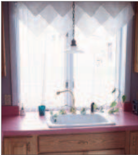
Figure 1. A projecting 2x12 "box" provides the structure for this small bay window. The counter extends flush right to the window unit.
