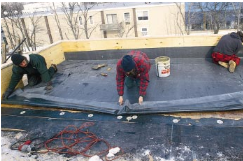
Figure 2. After the adhesive has tacked up, workers roll the EPDM into place (left). Wrinkles are smoothed out with a stiff bristle broom (right).
