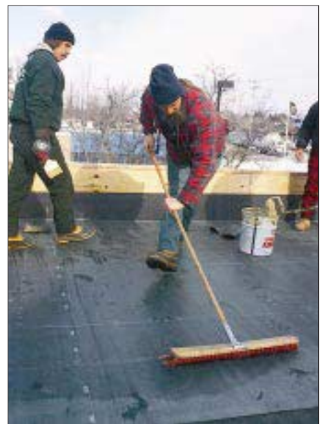
Figure 2. After the adhesive has tacked up, workers roll the EPDM into place (left). Wrinkles are smoothed out with a stiff bristle broom (right).
