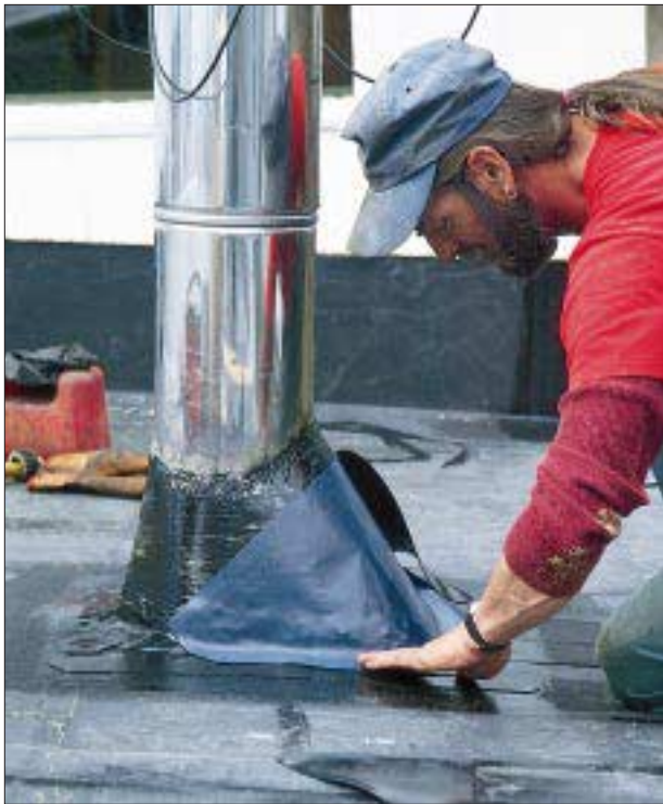
Figure 3. Uncured EPDM flashing membrane molds easily to roof penetrations like metal chimneys (left) and plumbing vent pipes. All flashing patches should be sealed with a fully glued double layer of EPDM (right).
