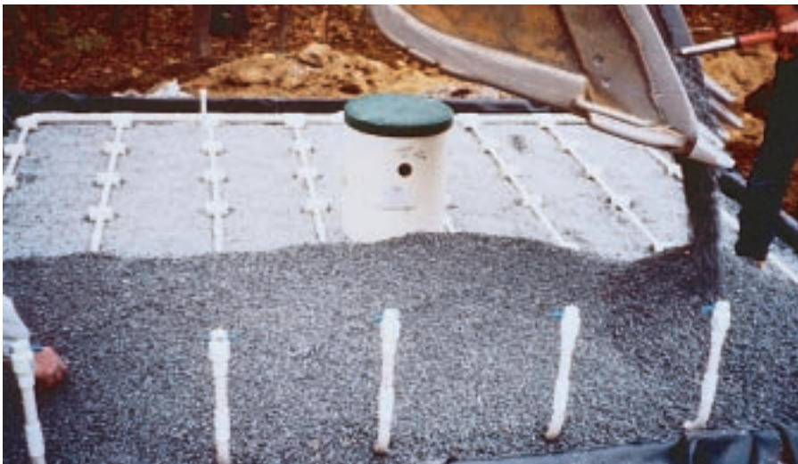
Figure 1. Construction of a sand filter begins with a pressure-treated wood box lined with tough plastic (see photo, page 36), with an optional pump chamber in the center. A foot-deep base layer of gravel is topped by a 2-foot layer of clean sand. Another foot-deep gravel layer supports and covers the grid of emitter pipes (left).
