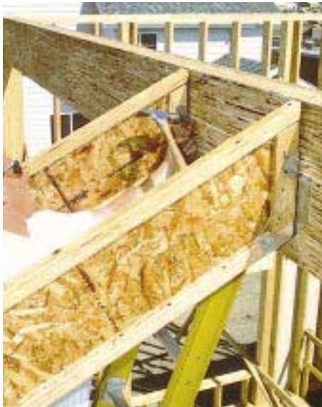
Figure 1. Sloped-seat hangers can be adjusted in the field to match the slope of the roof. These hangers require a plywood or lumber web stiffener on both sides of the I-joist to fill out the space between the hanger and the web.
