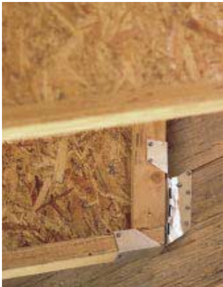
Figure 5. Sloped-seat hangers can be skewed up to 45° for hip and valley jack rafters. Compound cuts are not necessary; only the plumb cut needs to be made.
