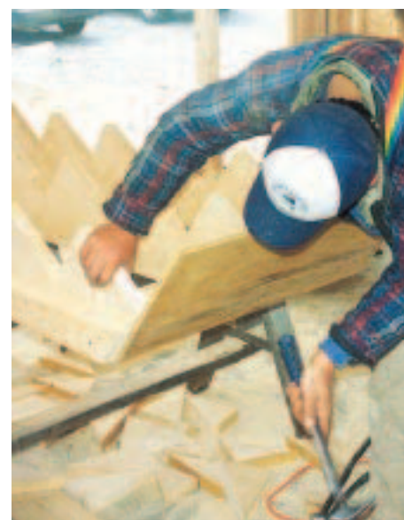
Figure 5. The author attaches a gusset and one temporary tread to hold his stringer assembly together. He nails the gusset to the second-floor framing to hold the assembly securely in place.
