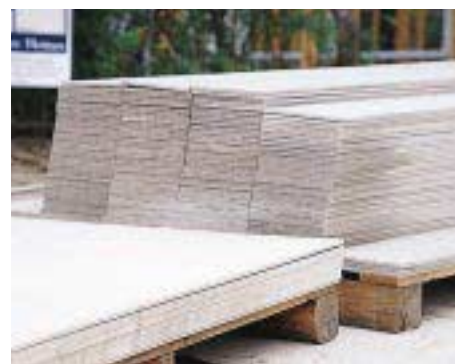
Figure 8. Dark rainwater stains on the end of this pallet of lap siding show how fiber cement absorbs moisture. As with masonry, the moisture doesn't hurt the material, but it should be allowed to dry before painting.
