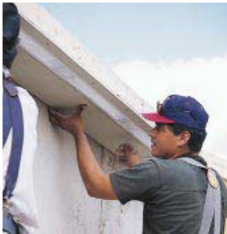
Figure 7. One problem with fiber-cement soffit is that it's hard to nail to. Tamlyn's Snapvent installs without fasteners, providing soffit ventilation while covering the fuzzy, ripped edges of the fiber-cement soffit.
