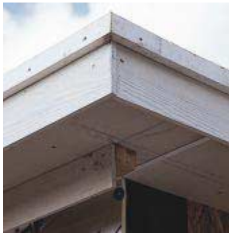
Figure 6. The frieze, soffit, and fascia on this house are made from fiber-cement, but the uppermost piece of trim is spruce. Builders often find themselves mixing wood and wood-based materials with fiber-cement, because fiber-cement does not yet come in a \frac{3}{4} -inch-thick size.
