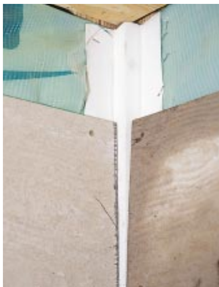
Figure 4. Tamlyn's vinyl inside corner trims are designed specifically for use with fiber-cement lap siding. Once painted, they look just like wood.
