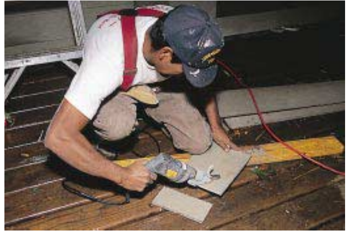
Figure 2. Snapper Lite shears work like motorized tin snips to make straight and curved cuts in fiber-cement without producing dust. The shears are slower than a circular saw but, claims the manufacturer, are cheaper to run than a saw.
