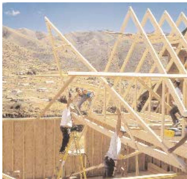
The SpaceMaker Truss , a ready-to-assemble roof framing system, uses TimberStrand LSL components. Truss parts are precut, notched, and predrilled for bolted connections. Hardware is included in the delivered package, which the manufacturer claims can be assembled with a socket wrench.
