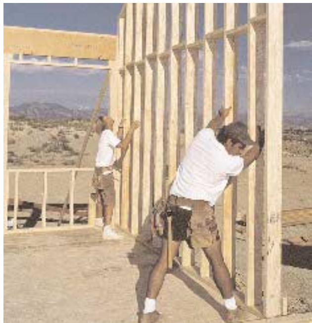
TimberStrand studs are an attractive alternative to dimension lumber for tall walls or where absolute straightness is an issue. But be prepared to pay a premium.
