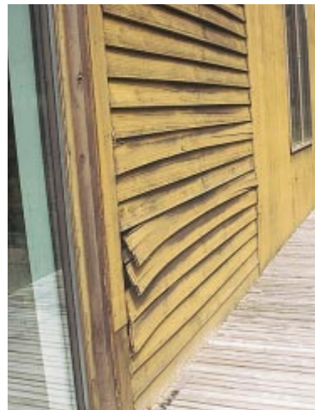
Figure 1. Years of sun and rain on the south-facing gable-end of this 17-year-old house (left) had caused delamination in the rough-textured T1-11 cladding (middle). Clapboards in the central feature strip had also cupped badly, exposing the underlying structure to moisture damage.
