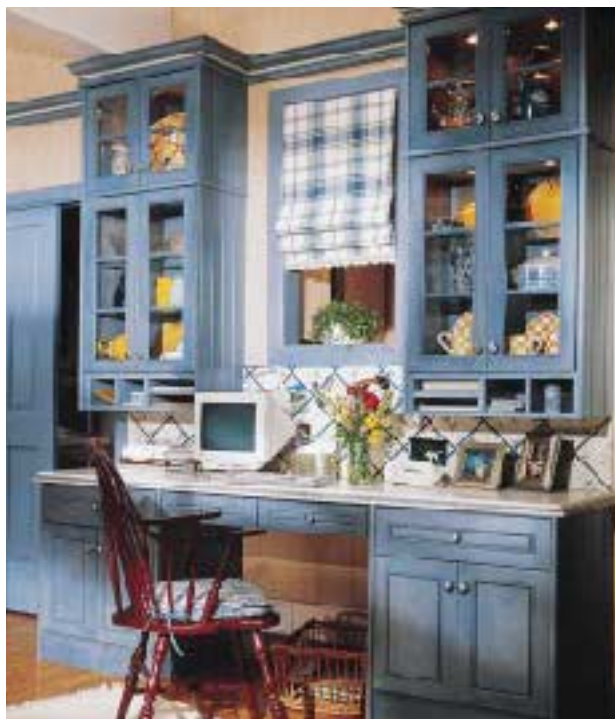
Figure 1. Extending a cabinet-top crown molding onto the adjacent walls integrates the cabinets into the overall design of the room (left). A crown molding can also be incorporated into a lighting soffit (above).
