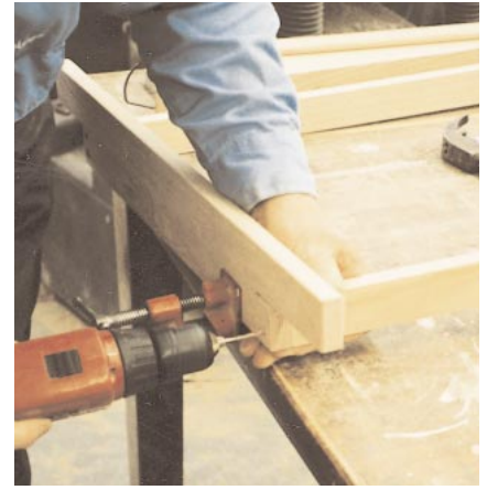
Figure 4. While the head trim assemblies are drying, the author assembles the jamb extension “boxes” using wood screws.
