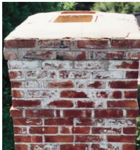
Figure 3. Flue liners should project at least 3 inches above the crown. Here, a thin crown and recessed flue liners caused this chimney crown to leak. As the water worked its way out of the chimney and evaporated, soluble salts remained behind, leaving a whitish stain called efflorescence.
