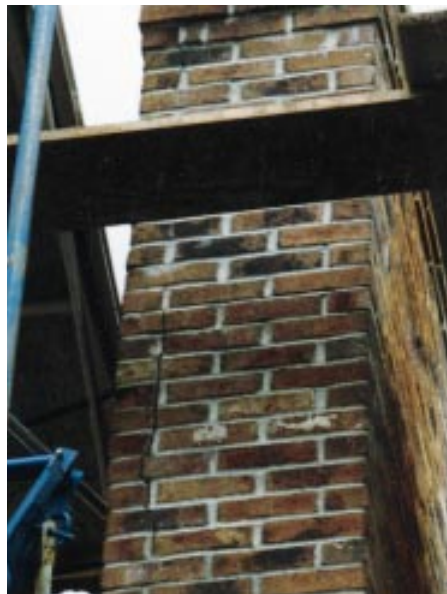
Figure 5. The code-required air space between the flue liners and the chimney walls allows the liners to expand and contract freely. In this chimney, the void between the bricks and the flue liners was filled solid with mortar, and resulted in a 7-foot-long crack when the liners expanded.
