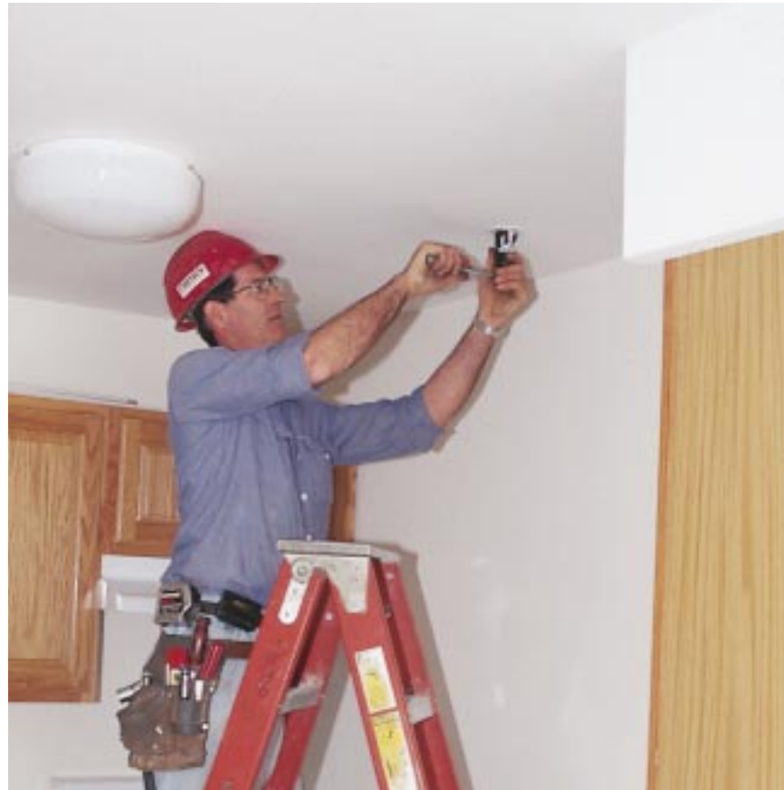
An installer uses a special wrench to mount a sprinkler head.
