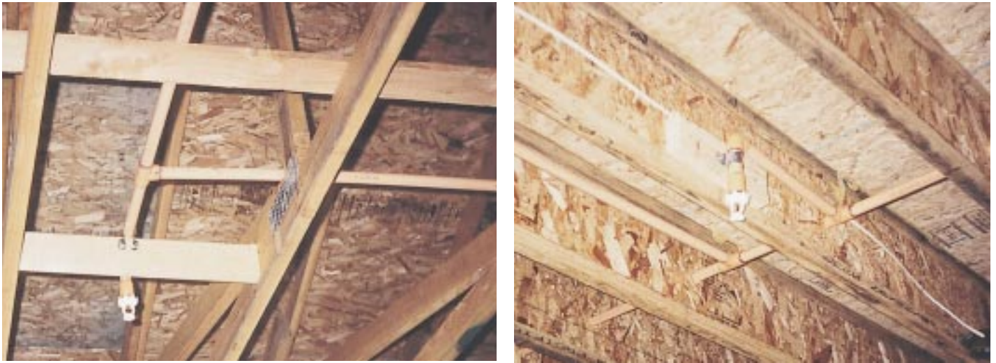
Figure 3. CPVC pipe must be properly blocked and strapped to prevent deformation under pressure.
