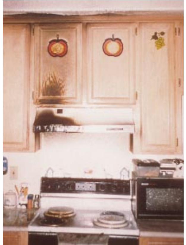
Figure 1. Sprinklers make a difference. A fire that started in a bathroom wastebasket spread quickly, causing $75,000 in damage (above); no sprinkler was installed. By contrast fire in a kitchen exhaust hood (right) was doused with a single sprinkler head, leaving $600 in damages.
