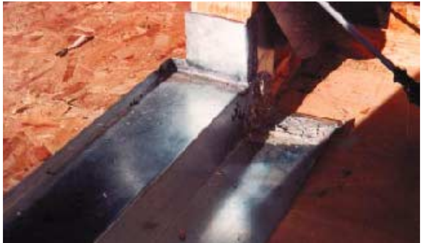
Figure 2. For doors installed over wood subfloors, the author uses a soldered metal pan at the sill, making sure the metal deck-to-wall flashing overlaps the side flanges and that the flashing paper around the opening is properly layered. All doors should be securely shimmed and nailed through the jambs to prevent cracks in the stucco from door movement.
