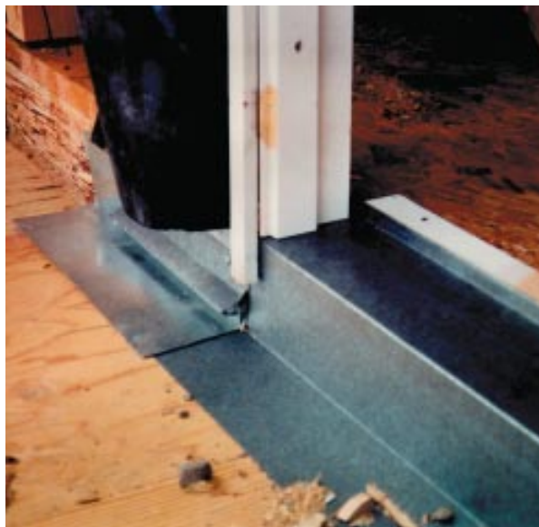
Figure 2. For doors installed over wood subfloors, the author uses a soldered metal pan at the sill, making sure the metal deck-to-wall flashing overlaps the side flanges and that the flashing paper around the opening is properly layered. All doors should be securely shimmed and nailed through the jambs to prevent cracks in the stucco from door movement.
