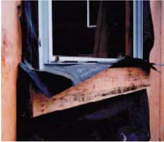
Figure 3. Flashing paper should be used behind wood or foam plant-ons used to trim openings. The plant-ons should be completely wrapped with flashing paper, which must also be properly woven into each course of lath paper for proper drainage.
