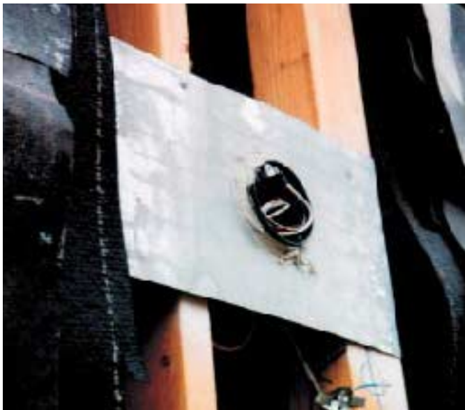
Figure 4. To flash wall penetrations, the author uses a two-piece sheet-metal collar (illustration), which is caulked to the fixture, then overlapped with flashing paper. A one-piece collar works well when the fixture falls in the center of a stud bay (photo, left). The integral flanges on attic and exhaust vents provide enough support for the stucco, but should still be caulked and carefully overlapped with flashing paper (photo, right).
