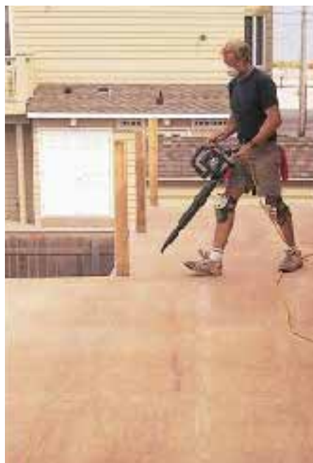
Figure 10. After the base coat has dried, sandpaper is used to knock down edges and rough up the whole surface to improve bonding with the finish coat (above). Brooms and leaf blowers are used to remove excess particles from the surface before applying the gel coat finish (left).
