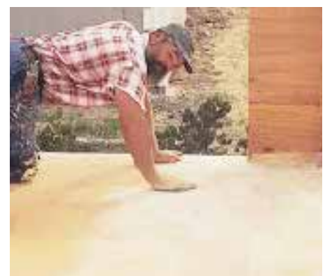
Figure 10. After the base coat has dried, sandpaper is used to knock down edges and rough up the whole surface to improve bonding with the finish coat (above). Brooms and leaf blowers are used to remove excess particles from the surface before applying the gel coat finish (left).
