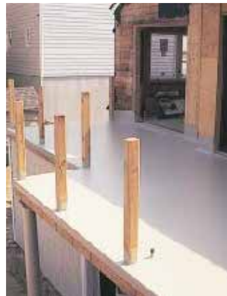
Figure 11. Tinted gel coat is applied first at edges and penetrations (left), then on the main deck (middle), using short-nap paint rollers. The final product cures in about 30 hours and looks much like the surface of a fiberglass tub (right).
