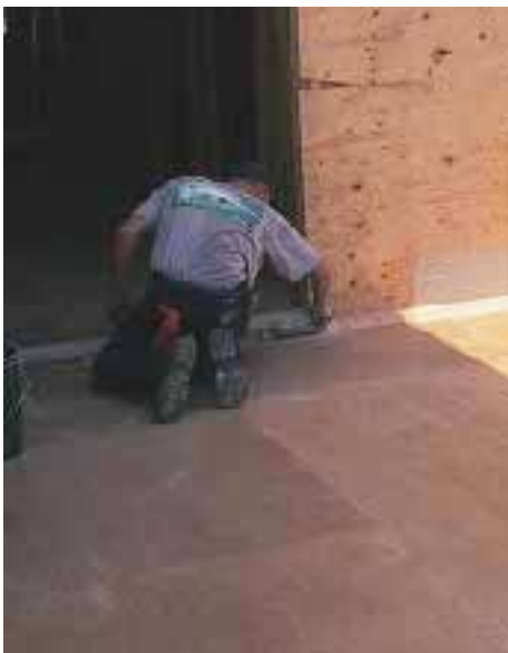
Figure 11. Tinted gel coat is applied first at edges and penetrations (left), then on the main deck (middle), using short-nap paint rollers. The final product cures in about 30 hours and looks much like the surface of a fiberglass tub (right).
