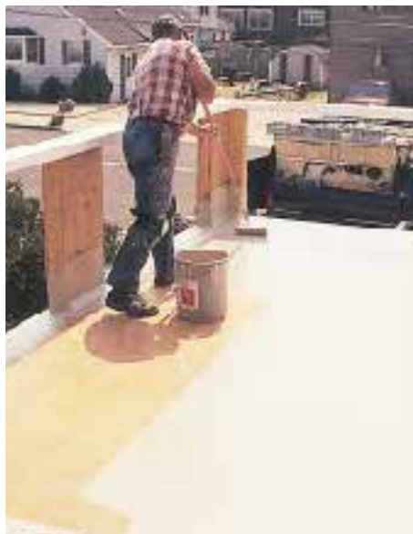
Figure 11. Tinted gel coat is applied first at edges and penetrations (left), then on the main deck (middle), using short-nap paint rollers. The final product cures in about 30 hours and looks much like the surface of a fiberglass tub (right).
