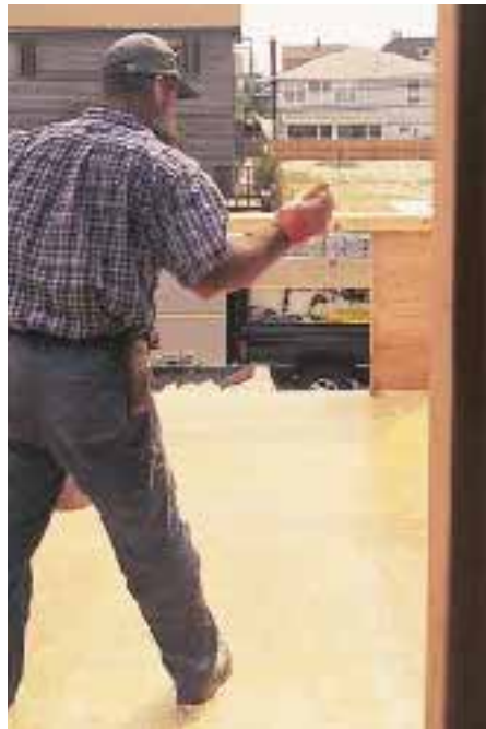
Figure 9. At the main deck, a bedding coat of fresh resin is applied in 4-foot bands using a short-nap paint roller, covered with a full-width sheet of fiberglass mat, then rolled again (above). Clean sand is then spread over the still wet mat to provide a nonskid surface (left).
