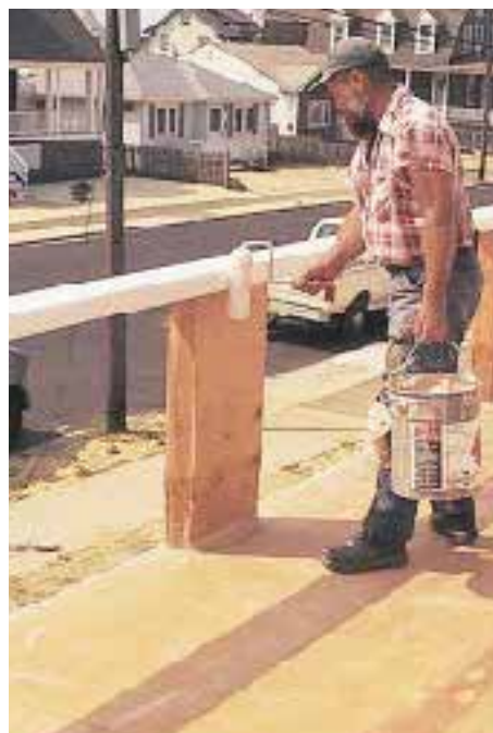
Figure 12. On this job, the wood railings were also flashed with fiberglass mat (left), then finished with white gel coat to contrast with the deck color (right).
