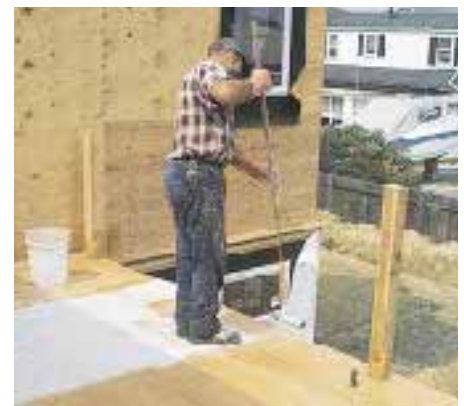
Figure 9. At the main deck, a bedding coat of fresh resin is applied in 4-foot bands using a short-nap paint roller, covered with a full-width sheet of fiberglass mat, then rolled again (above). Clean sand is then spread over the still wet mat to provide a nonskid surface (left).
