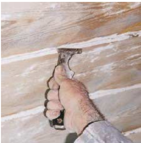
Figure 6. The author uses carbide scrapers (above) and painter's picks (right) to remove paint and caulk buildup at the bottom of clapboards. This ensures good ventilation behind the siding.
