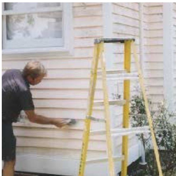
Figure 10. The final top coat is always brushed on, trim-work first.
