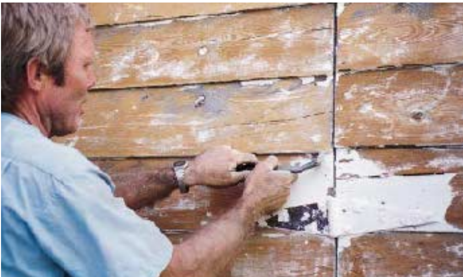
Figure 6. The author uses carbide scrapers (above) and painter's picks (right) to remove paint and caulk buildup at the bottom of clapboards. This ensures good ventilation behind the siding.
