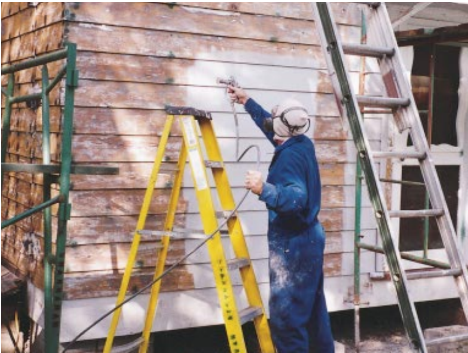
Figure 9. The oil-based primer is typically sprayed (unless neighboring houses are too close or the clients insist on brush and roller only). Note the treated nail heads, and how the author boxes out the work area (above). The author uses a Titan Epic 660 sprayer (right), which can handle unthinned paints without clogging.
