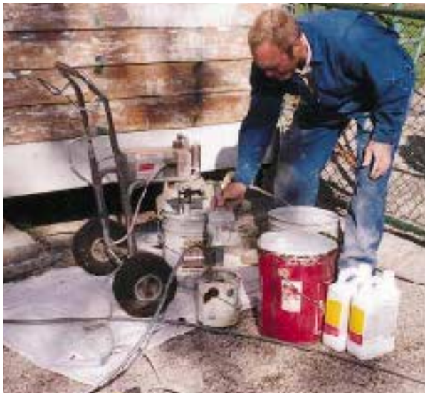
Figure 9. The oil-based primer is typically sprayed (unless neighboring houses are too close or the clients insist on brush and roller only). Note the treated nail heads, and how the author boxes out the work area (above). The author uses a Titan Epic 660 sprayer (right), which can handle unthinned paints without clogging.
