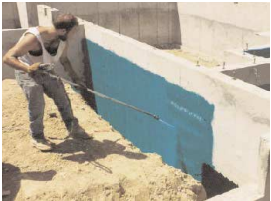
Figure 1. Spray-applied foundation membranes come in two main types — a distinctive green (or yellow) solvent-based rubber (top) and a water-based, polymer-enhanced asphalt (left).
