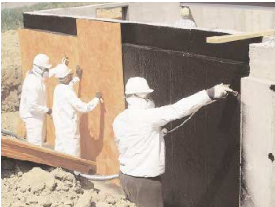
Figure 2. Spray-applied foundation systems typically include protective foam or fiberglass panels. These must be applied over the membrane to protect the coating from damage during backfilling and to help reduce hydrostatic pressure.
