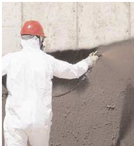
Figure 1. Spray-applied foundation membranes come in two main types — a distinctive green (or yellow) solvent-based rubber (top) and a water-based, polymer-enhanced asphalt (left).
