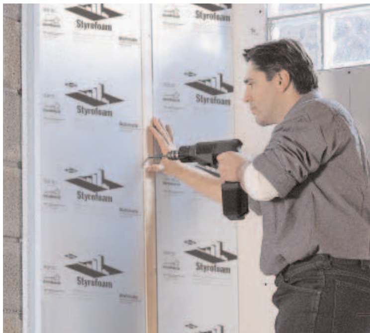
Figure 6. For interior basement insulation, wide shiplaps on some XPS boards accept furring strips, which can be fastened through the foam to poured concrete or masonry (left). Diversifoam's "CertiStud" EPS board has plywood furring strips bonded to the foam (above).
