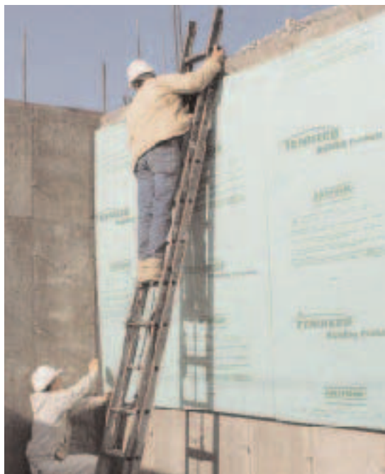
Figure 2. Because of its high resistance to moisture, XPS is the best material to use in wet locations or in contact with the ground. At foundations, a waterproofing membrane is still required, however, since water can still migrate through joints between sheets.
