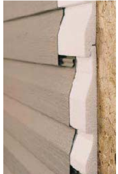
Figure 7. Some foam producers, such as Progressive Foam Products, mold EPS to match common vinyl siding profiles and accessories. However, not all such EPS moldings are approved by all siding manufacturers, and some siding companies will not warrant their products when installed over EPS.
