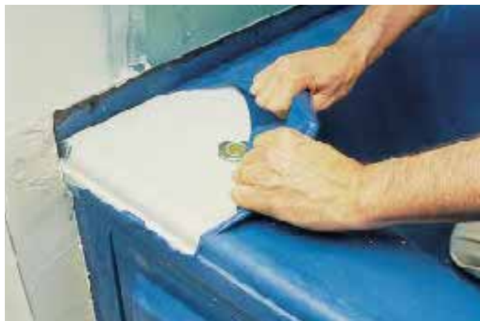
Figure 8. Liquid coatings that cure to form a rubbery film are a good way to protect vulnerable, irregular-shaped plastic and porcelain tub surfaces. Liquid Mask from ProTect is shown here.
