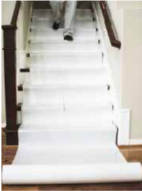
Figure 4. Self-adhesive films cover hard and soft floor surfaces to prevent scuffing and ground-in dirt. Floorliner (left) has a soft cotton backing, and can stay in place up to 120 days. Protection for carpets from Dust Door (right) keeps dirt on the surface for easy removal, and can be left in place for up to 45 days.
