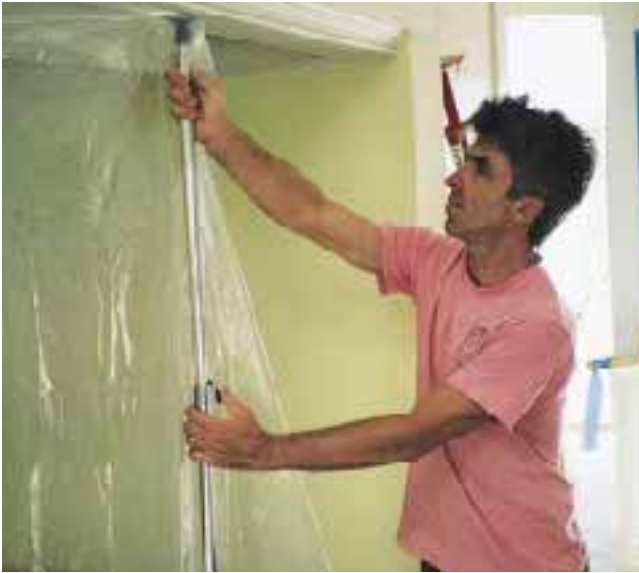
Figure 1. Telescoping Curtain Wall poles make short work of dust and paint spray containment in rooms with up to 12-foot ceiling heights.
