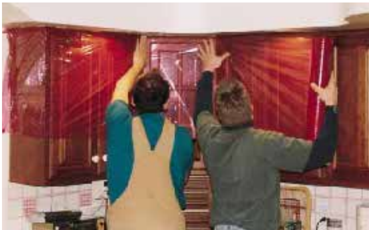
Figure 10. Static-clinging thin plastic films like Dust Door’s MultiUse Red or Poly-Tak’s Window Mask are excellent for protecting glazing or cabinets from paint splatters.
