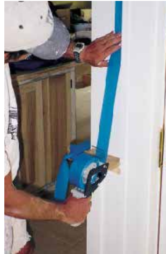
Figure 11. Masking tape goes on quickly and accurately with a dispenser. Use an easy-peel UV-resistant product like Shurtape for exposure up to 7 days.
