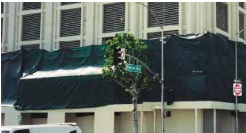
Figure 5. Rugged tarps serve many uses, including wind screening and dust containment. Nathan Kimmel's durable lightweight tarps are used widely in the plaster and stucco trades.
