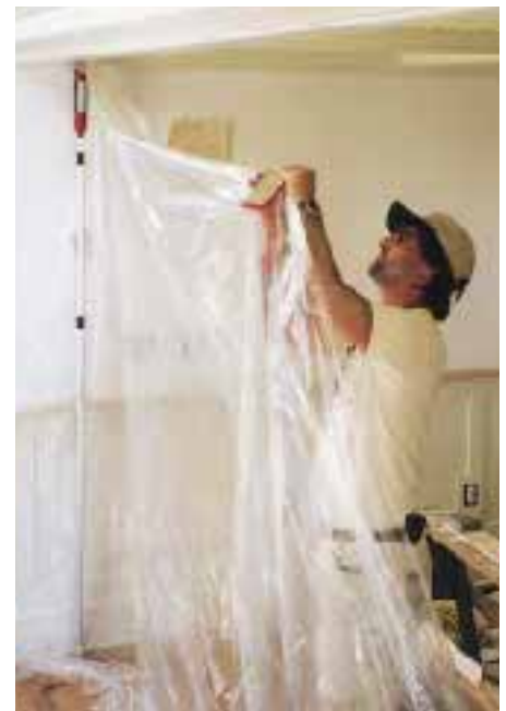
Figure 3. The standard telescoping pole from ZipWall has a 12-foot reach, adjusts easily, and compresses in place to allow the user to trap the bottom edge of the curtain.
