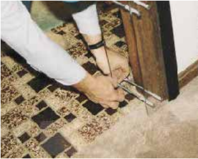
Figure 7. Dust Door's jamb protector (above) also provides a surface for mounting the dust curtain using Velcro (right).
