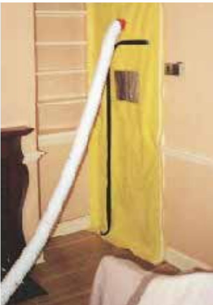
Figure 2. High-quality airtight components and exclusive features like the 4-inch exhaust-duct sleeve make it possible to create a negative-pressure work zone behind the Dust Door.
