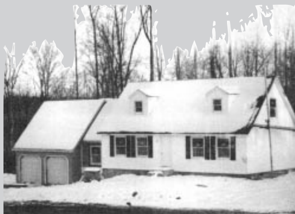
Cape Cod modulars sat under plastic (top) until a local roofing contractor could finish the roofs. Some units have a site-built breezeway and garage added as an option (bottom).
