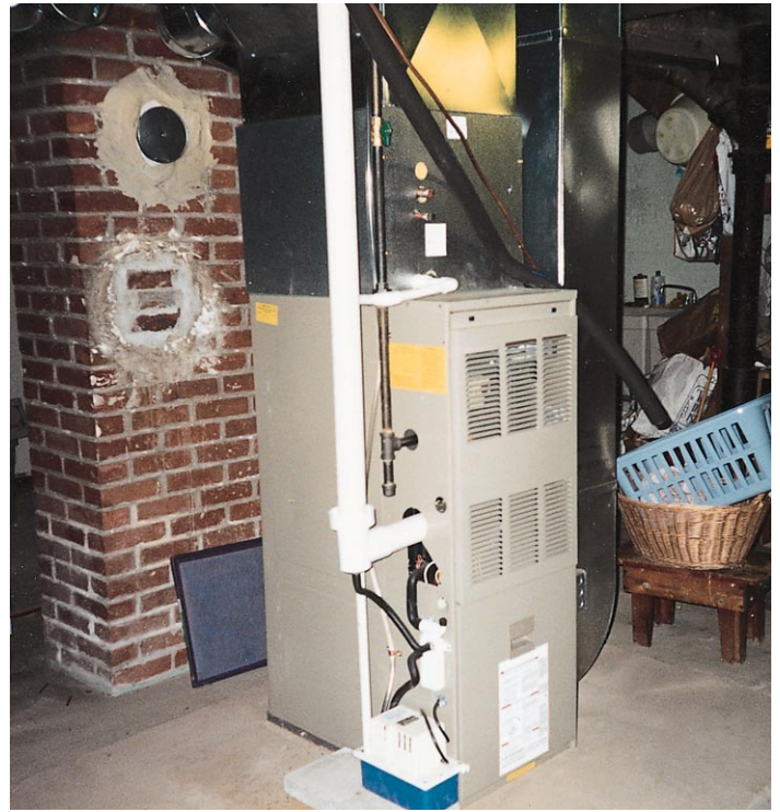
Figure 1. This standard-efficiency furnace (left) vents into an unprotected chimney on an outside wall. The poor draft has resulted in excessive flue gas condensation, which has corroded the galvanized flue pipe. Instead of repairing a damaged chimney, it is often less expensive to install a PVC-vented high-efficiency furnace (right).
