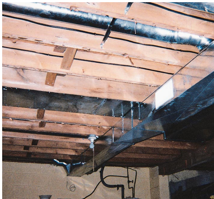
Figure 6. Trunk lines commonly step down to maintain air velocity. The capacity of the trunk at each step-down point must equal the capacity of all the branch runs that come after it.
