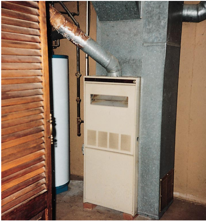
Figure 1. This standard-efficiency furnace (left) vents into an unprotected chimney on an outside wall. The poor draft has resulted in excessive flue gas condensation, which has corroded the galvanized flue pipe. Instead of repairing a damaged chimney, it is often less expensive to install a PVC-vented high-efficiency furnace (right).
